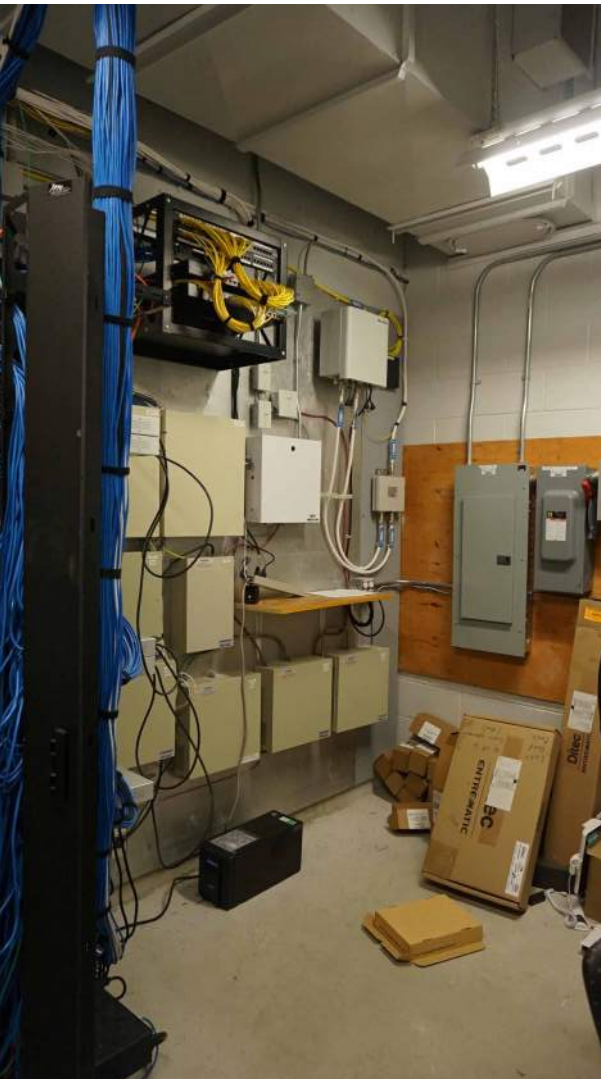
3 PHOTO #2 - DOOR ACCESS CONTROL PANELS SCALE: N.T.S.
