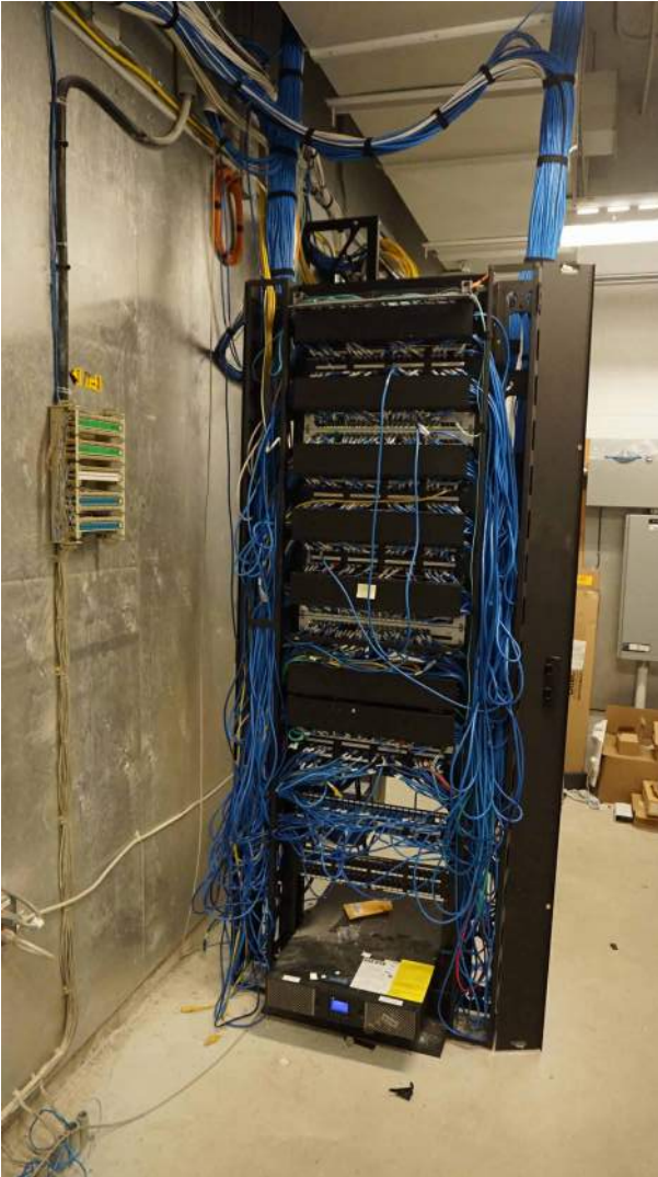
2 PHOTO #1 - IT RACK AND PATCH PANELS SCALE: N.T.S.
